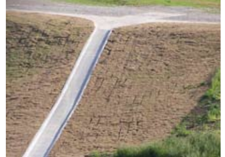
Sump erosion corrected
