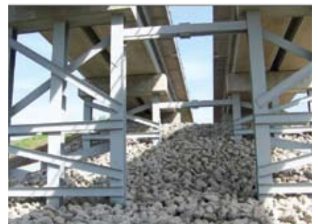
Levee erosion corrected
